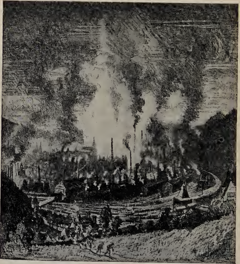
FIG. 126. THE MUNITION WORKS, LE CREUSOT, FRANCE
